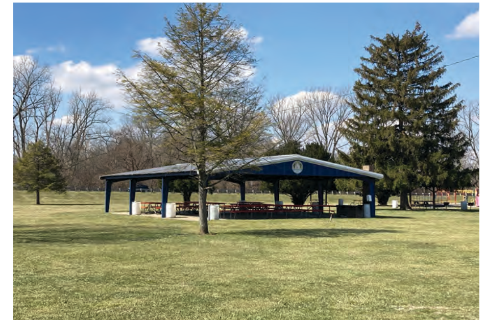
Community Park shelter
