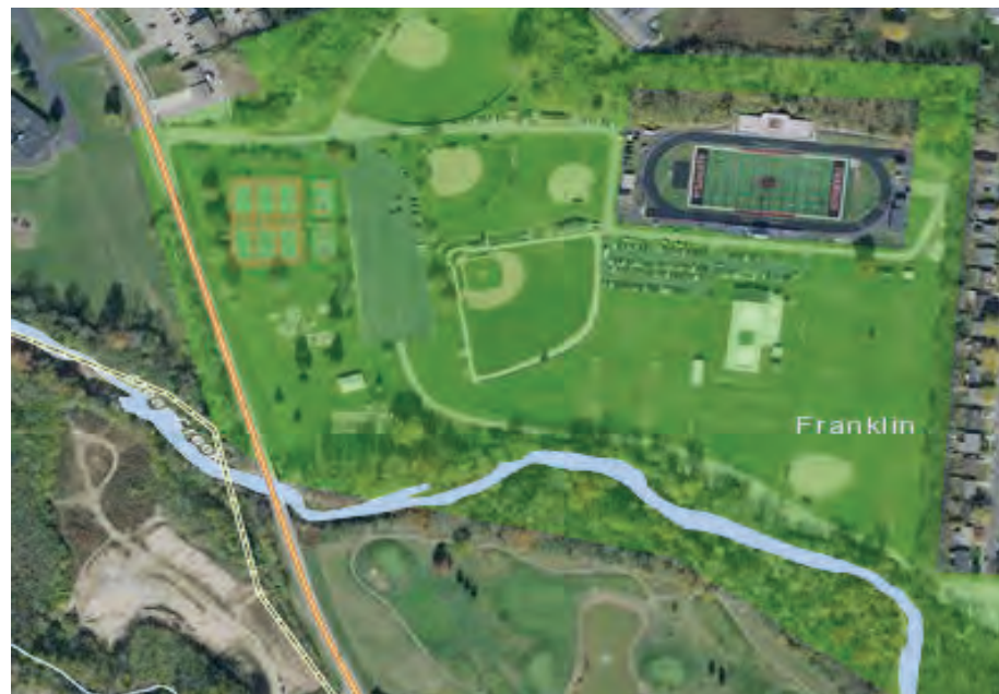
Community Park aerial view
