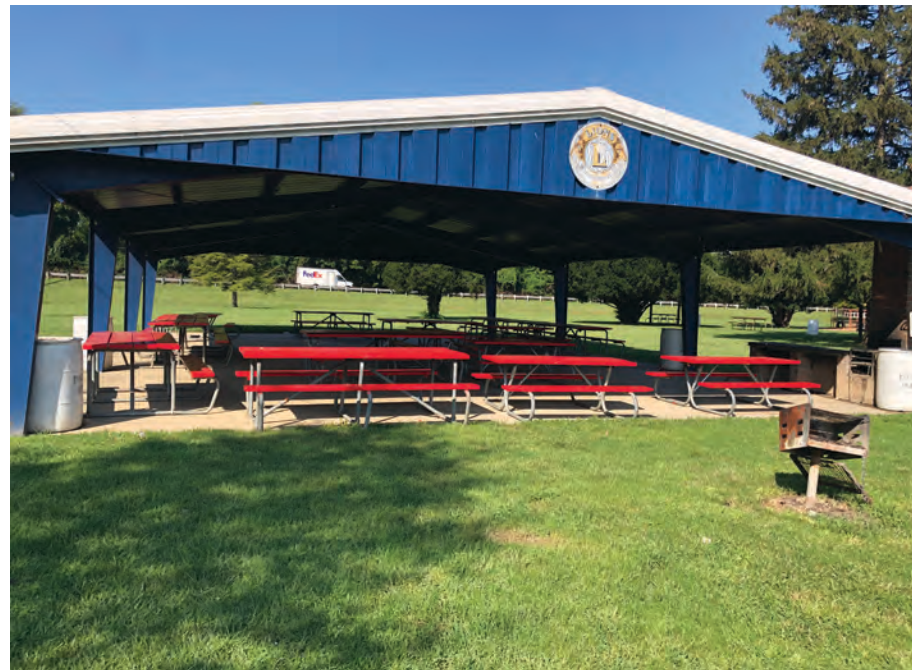
Community Park shelter
