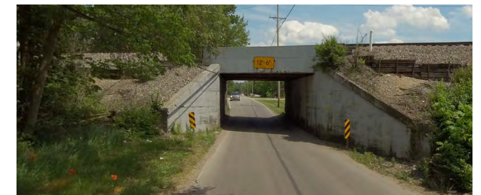
Railroad overpass along Franklin-Trenton Road
