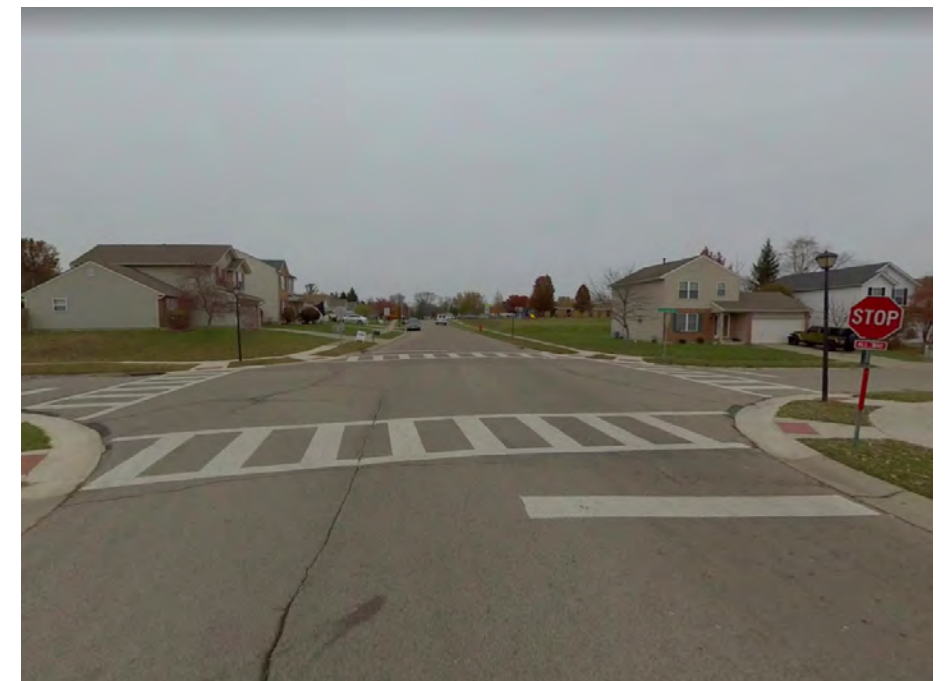
Residential intersection between Apache Street and Sherman Drive.
