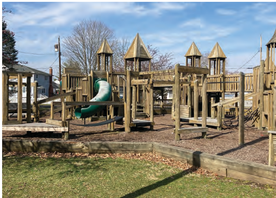
Community Park playground
